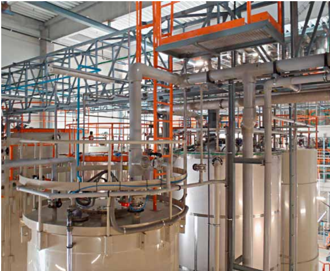
7 Network of tanks and pipelines inside the ReduDust building
