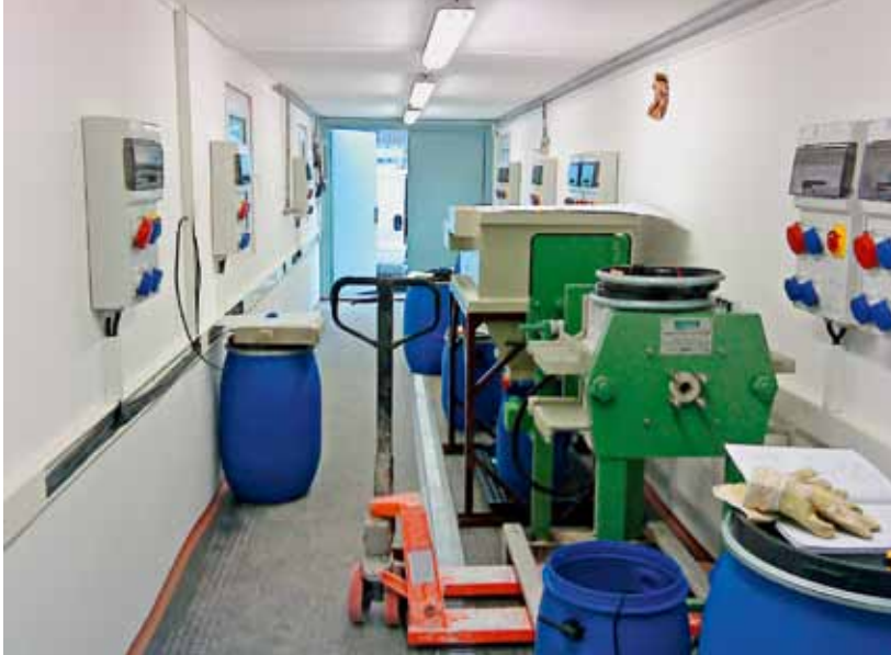
4 The process container of the 100 kg/day ReduDust pilot installation
