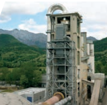
CEMENTIZILLO, Fanna Cement Plant
